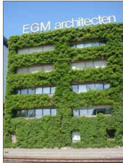
Figure 2.13 Left photograph detail example of a twining plant (Wisteria) against a façade with horizontal and vertical installed (grid) stainless steel rope system; Right photograph final result of the complete façade (Dordrecht, The Netherlands).
