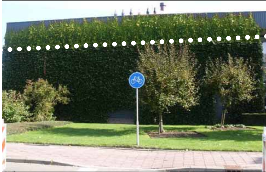
Figure 3.23a Maintenance an annual deficiency of green façades, above the dashed line has to be pruned each year to avoid that the shoots will grow over the roof, Photo Ashraf Mir.
