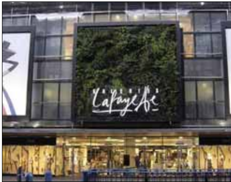
Figure 3.2a Left: Prefab growing system or living wall system created by Patrick Blanck (Berlin, Germany). 3.2b Right photo: Also artificial growing substrate panels; living wall concept of Cultilene Saint Gobain.
