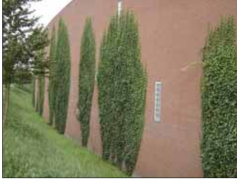
Figure 3.1a Left: rooted into the ground directly against the façade, 3.1b Right: rooted into the ground indirectly against the façade (photo Hoek hoveniers).
