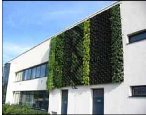
Figure 3.2a Left: Prefab growing system or living wall system created by Patrick Blanck (Berlin, Germany). 3.2b Right photo: Also artificial growing substrate panels; living wall concept of Cultilene Saint Gobain.
