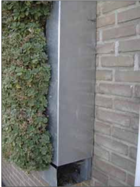
Figure 5.13 Living wall system (Fytowall) attached to a façade. One can see clearly the well finished edge. Due to this detailing one can interpret the existing cavity between panel and masonry as a "un ventilated" air layer.
