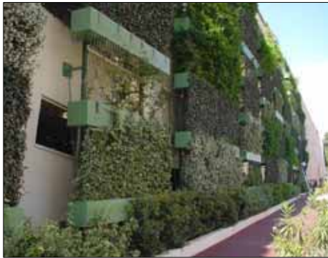
Figure 3.3a Left: not rooted into the ground; indirectly against the façade (Monaco). 3.3b Right photo: Detail of a planter boxes system against façade (photos Huib Sneep).
