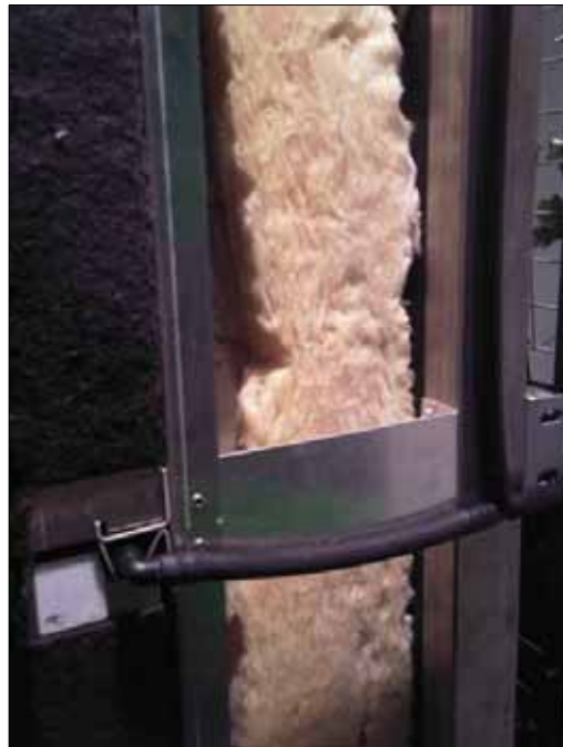
Figure 5.12 Modular living wall system (LWS); space between façade and panel filled with "extra" insulation material. Very suitable principle for retrofitting of older buildings that are less insulated.
