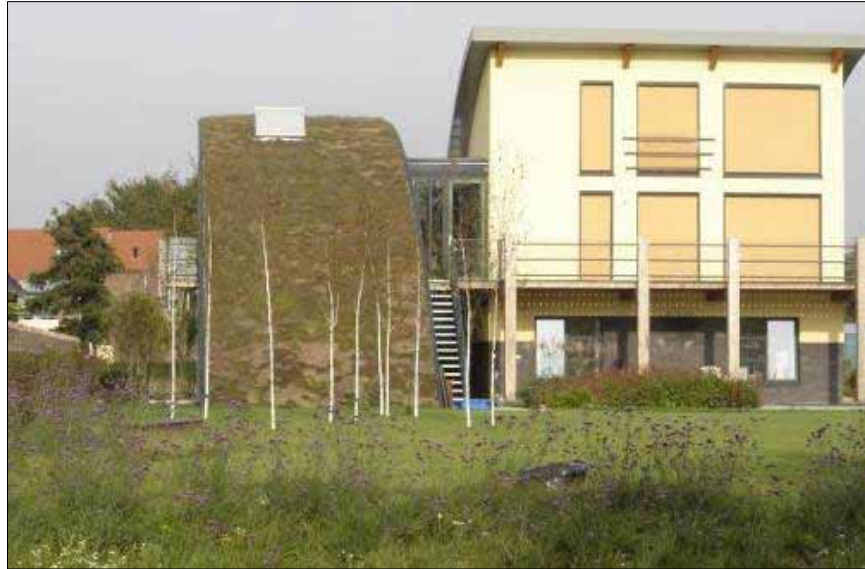
Figure 2.8 Modern version of a (Sedum planted) green roof. (Texel, The Netherlands.)
