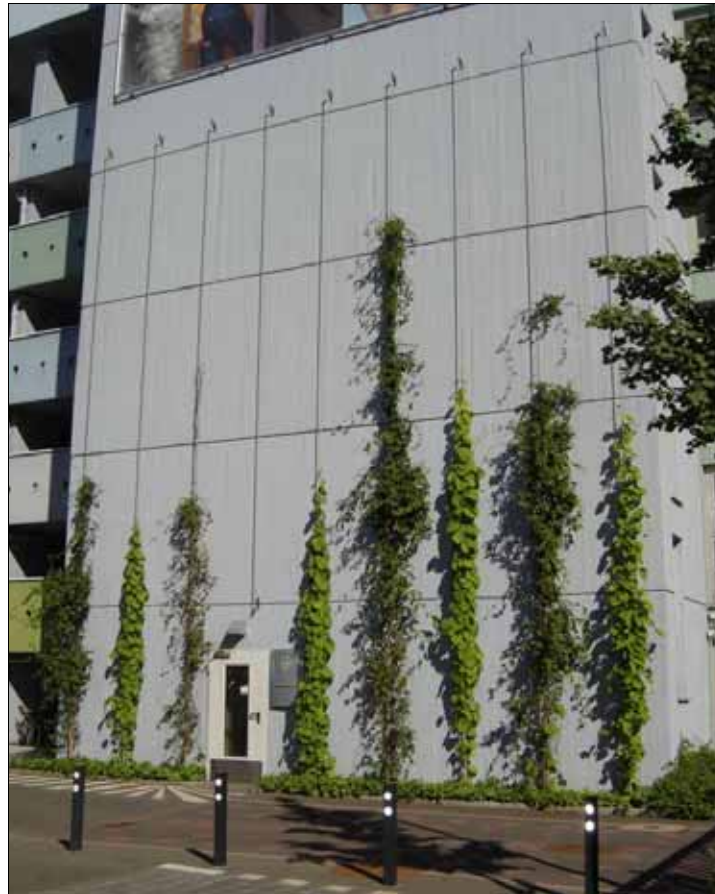
Figure 2.14 Example of twining plants (Aristolochia and Wisteria) against a façade using a vertical stainless steel rope system (Berlin, Germany).
