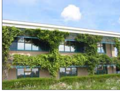
Figure 3.1a Left: rooted into the ground directly against the façade, 3.1b Right: rooted into the ground indirectly against the façade (photo Hoek hoveniers).
