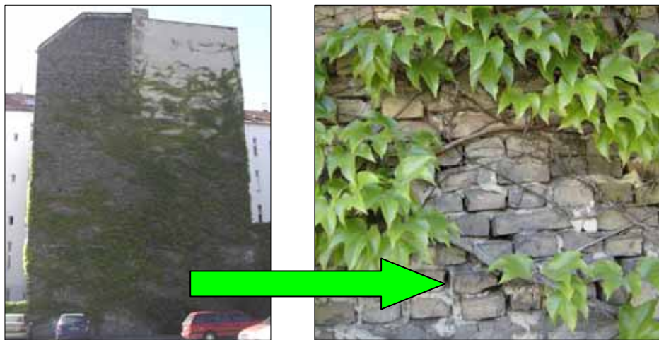
Figure 3.20 An old façade (brick wall with porous lime stone mortar joints) in the inner city of Berlin partially covered with Boston ivy ( Parthenocissus ). Although not advisable to use a direct
