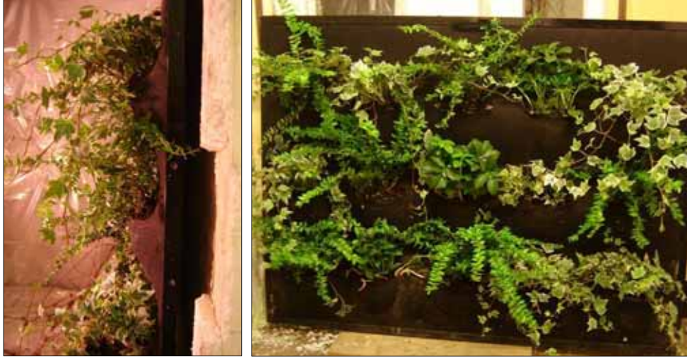
Figure 5.83 Several thin layers of felt are used to let grow plants. From the PVC sheet the layers are: 2 mm of synthetic textile felt, 5 mm felt of non woven fabric made of restructured recycled fibres, 0.1 mm perforated plastic sheet and 2 mm of black synthetic textile felt. The plants are planted in created pockets by cutting the outer felt layer (2mm sheet of black synthetic textile). Plants used are Hedera helix and Pachysandra.
