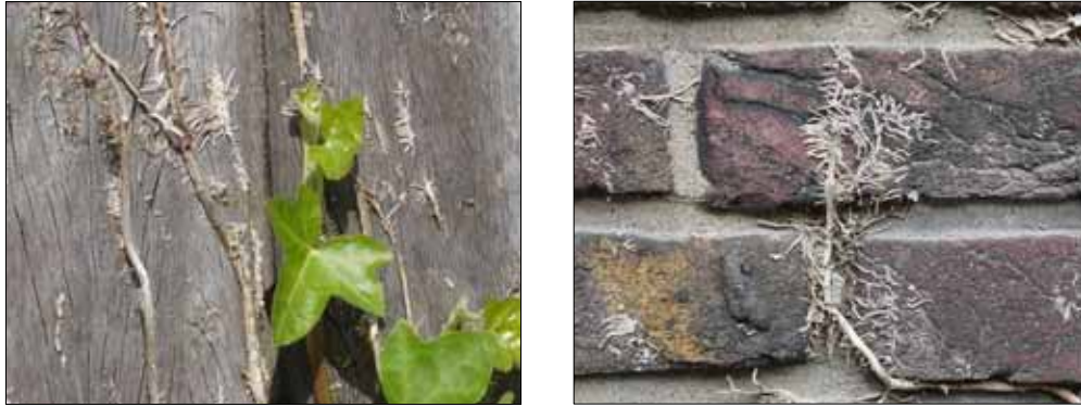
Figure 2.11 Aerial roots of Common ivy ( Hedera helix ) on wood and masonry.
