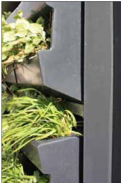
Figure 5.15 Right; modular living wall system (planter boxes) against the façade with closed edges to ensure a stagnant air layer between modules and façade.
