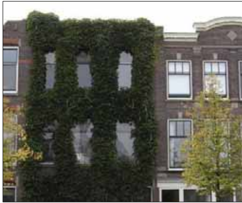
Figure 3.14 Boston ivy (Parthenocissus) rooted in the soil and applied directly against the façade in Delft summer 2009.
