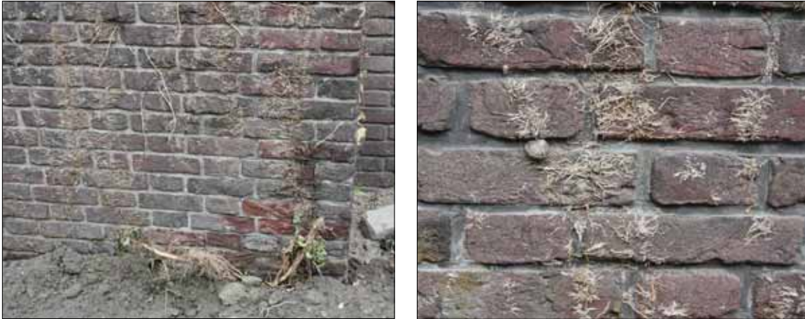
Figure 3.5: left, sucker root structure remains after removing the plants ( Hedera helix ) from the wall; right, biodiversity due to sucker root structures.
