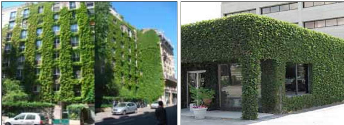
Figure 2.3a: different green façades with self-climbing plants directly to the wall (source: left, www.groenedaken.mht and right, www.greenscreen.com ).
