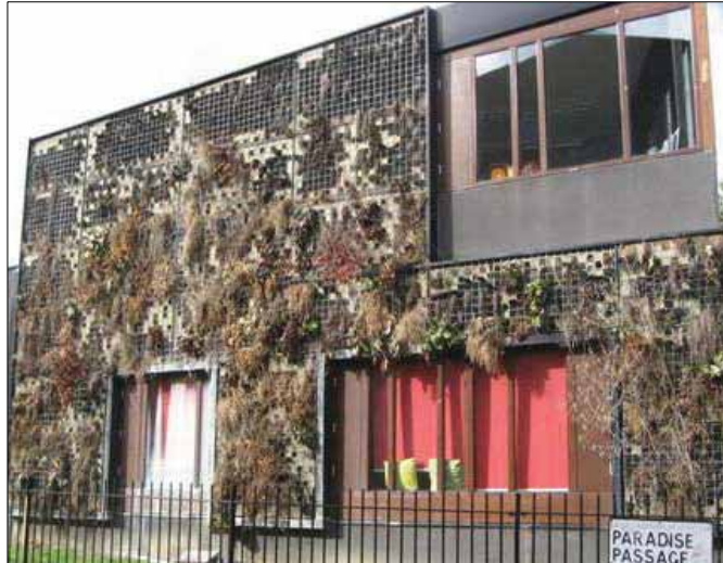
Figure 3.7: (a) bare parts on a felt layer system with died plants (source: Middellie, 2009); (b) torn pockets, water leakage and degradation of the substrate on a panel of felt layer system (source: Peters, 2011).
