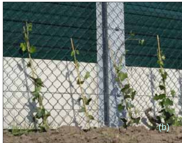
Figure 2.8: (a) mounting supporting structure on the Wall (source: www.greenscreen.com ); (b) applying green on supporting structure (netting system).
