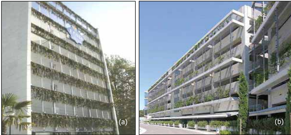
Figure 2.12: plants from intermediate planter boxes with supporting structure; (a) a hotel building (hanging system) (source: www.wallfore.eu ); (b) a multi-level parking structure (source: www.greenscreen.com ).
