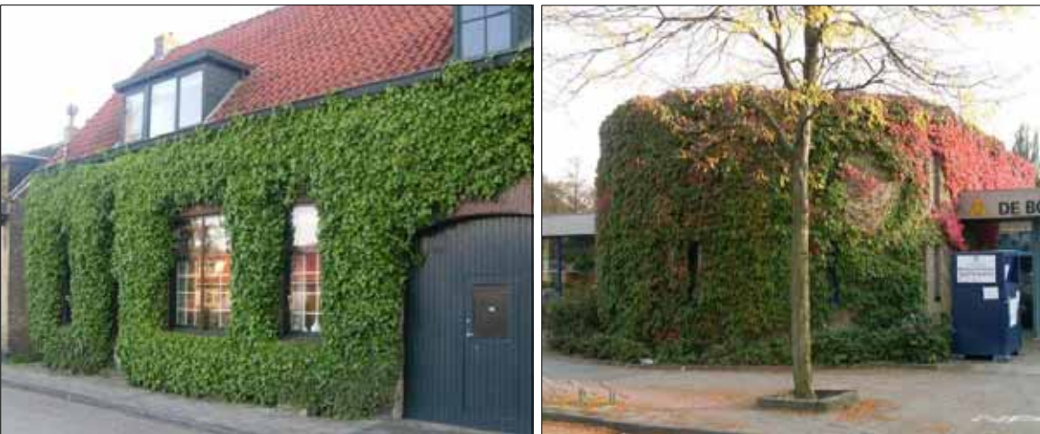
Figure 2.3b: different green façades with self-climbing plants directly to the wall; left, Dordrecht; right library building in Sliedrecht.
