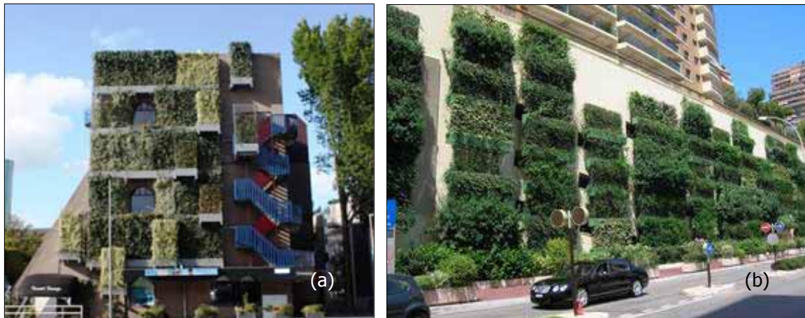
Figure 2.13: plants from intermediate planter boxes with supporting structure; (a) a multi-level building in Rotterdam; (b) a multi-level hotel building in Monaco; (source: www.greenwavesystems.eu/verticaletuinen ).
