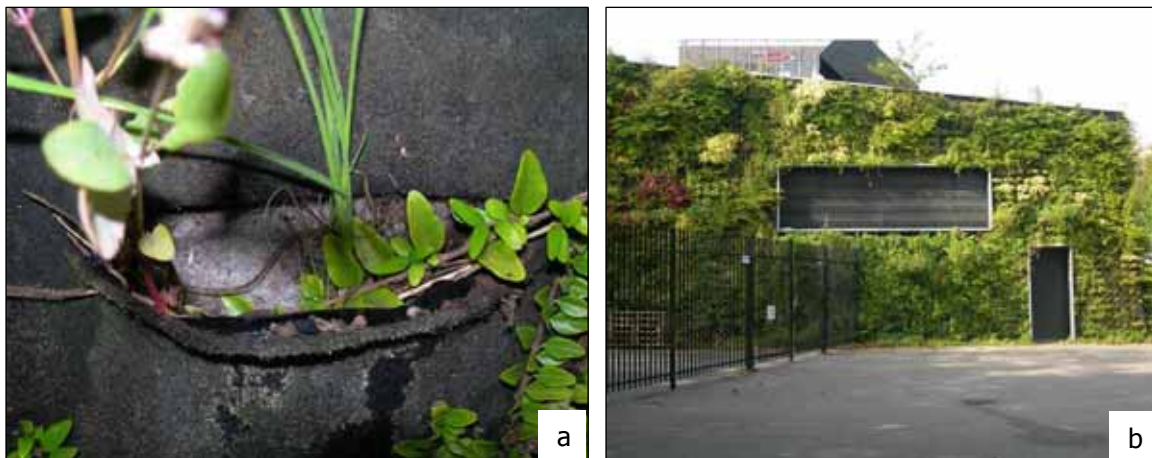
Figure 2.35: (a) plant bag from a façade of Mercator sport plaza (Amsterdam); (b) the building of Mercator sport plaza covered with LWS based on felt layers (source: www.deGroenestad.nl ).
