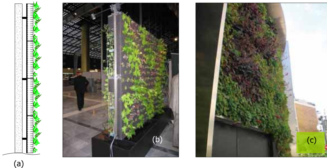
Figure 2.28: (a) principle of mineral wool based living wall system (wallflore); (b) mobile panel wallflore living wall system (source: www.wallflore.eu ); (c) wallflore living wall system applied outdoor.
