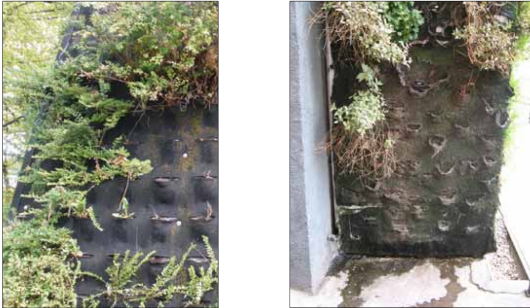
Figure 3.7: (a) bare parts on a felt layer system with died plants (source: Middellie, 2009); (b) torn pockets, water leakage and degradation of the substrate on a panel of felt layer system (source: Peters, 2011).
