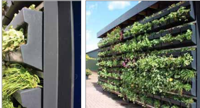
Figure 2.22: left, planter boxes with various plants in it (side view); right, living wall system with planter boxes including various plants.
