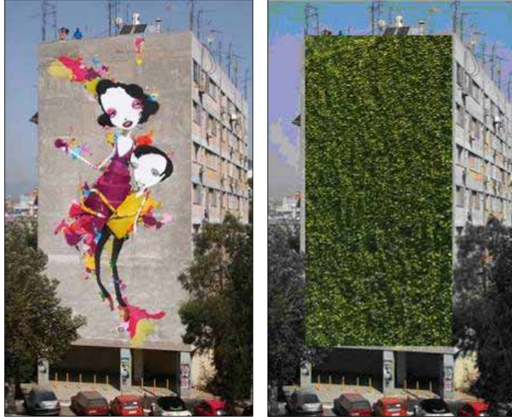
Figure 3.3: the façade of a building; left, before applying green and right, after applying green on it. (source : http://pileofphotos.com/pics/287910building_graffiti_01.jpg ).
