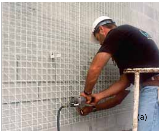
Figure 2.8: (a) mounting supporting structure on the Wall (source: www.greenscreen.com ); (b) applying green on supporting structure (netting system).
